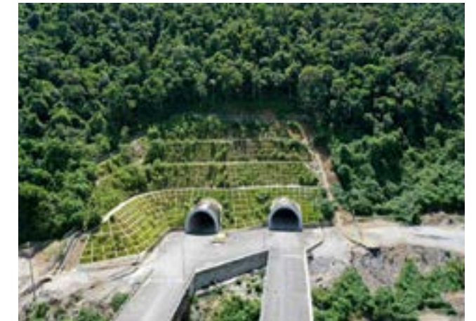
Hầm đôi Mũi Trâu - Cao tốc La Sơn - Túy Loan Double Tunnel of Mui Trau on La Son - Tuy Loan Expressway
