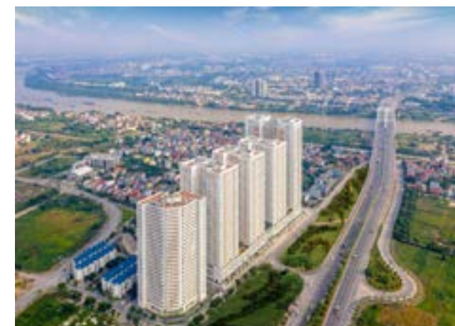
Nhà máy xử lý nước thải KĐT EuroWindow River Park Water treatment factory - EuroWindow River Park urban area
